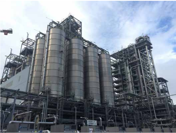
HDPE: Blending Silos. Punch clearance ongoing
