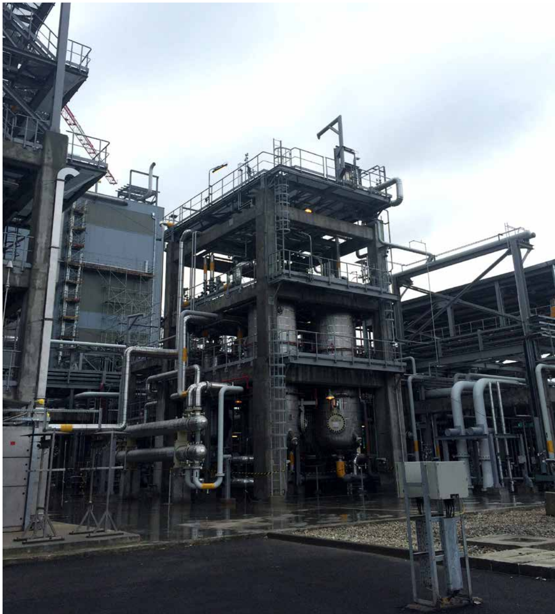
HDPE: Ethylene Treatment. Punch clearance in progress
