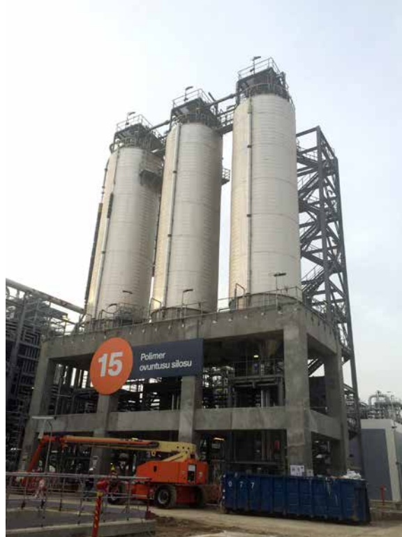
PP/U&O: PP Dry section / Powder Silos. Pre-commissioning activities in progress
