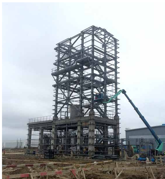
HDPE: Catalyst Activation. SS erection in progress
