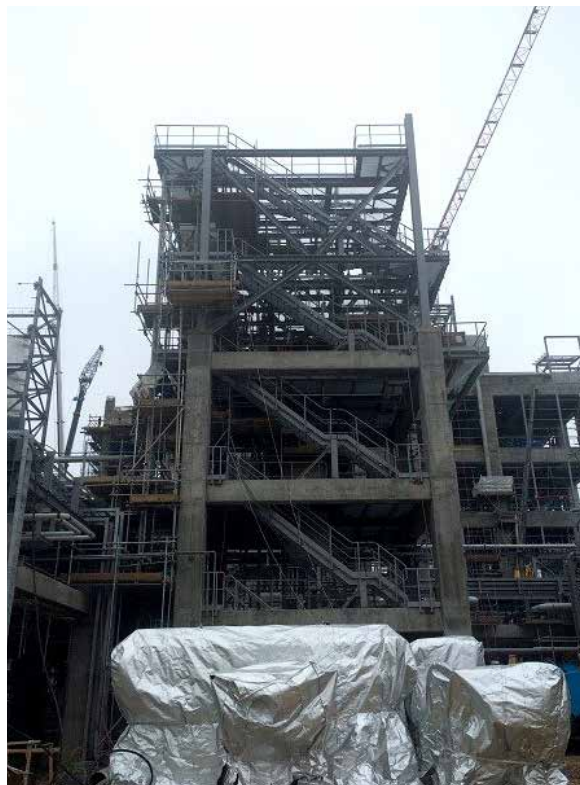
HDPE: Low Pressure Solvent Recovery. Instrument installation and cabling completed
