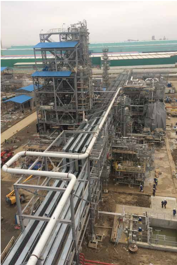
PP/U&O: PP- Wet section / Polymerization. Equipment testing in progress. Installation of electrical instrumentation ongoing. Piping test in progress. Branch cable tray installation in progress
