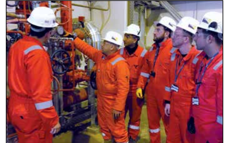
On-the-job training sessions at the SOCAR Polymer plant site
