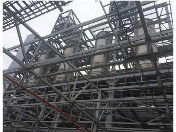
HDPE: Bagging & Packing. SS and cladding erection in progress. Equipment installation ongoing
