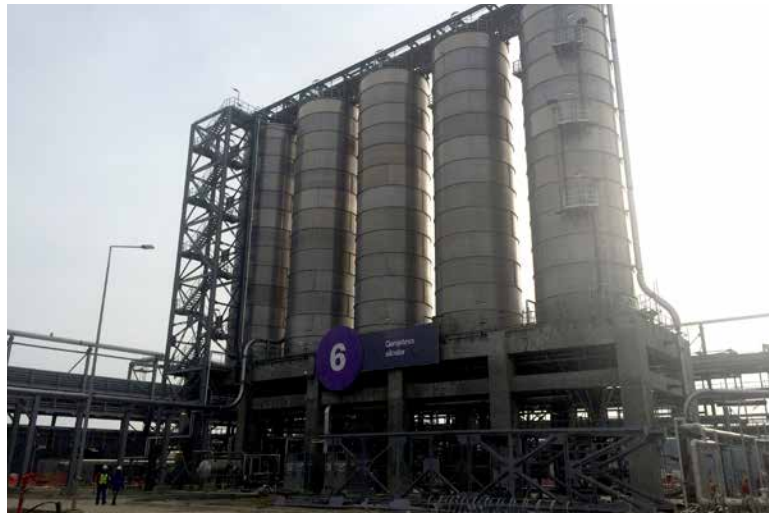
PP/U&O: Homogenization / Blender Silos. Pre-commissioning activities in progress
