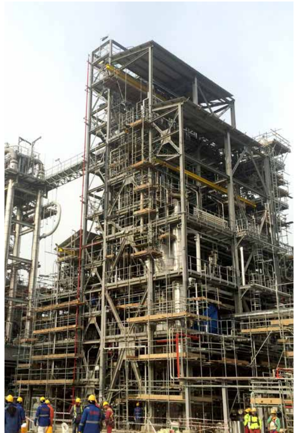
PP/U&O: PP- Wet section / Polymerization. Equipment testing in progress. Installation of electrical instrumentation ongoing. Piping test in progress. Branch cable tray installation in progress
