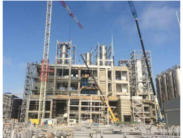
HDPE: Extrusion Structure. RCC works completed. SS and piping erection in progress. Junction box and sandwich panel installation in progress
